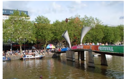
Bridge in Bristol Harbourside
